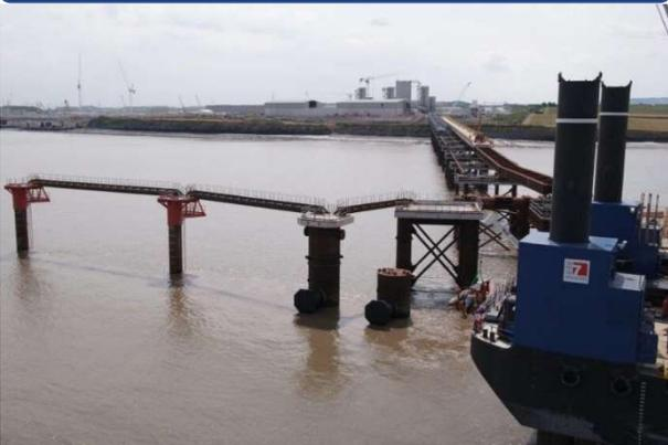
Construction of a 500 metre long jetty to allow materials for the local project to be delivered by sea was required. This would keep many hundreds of lorries off the local roads, reducing carbon emissions and disturbances to the local communities.
